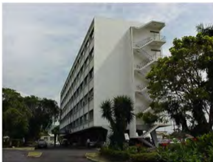
Figure 5: Ministry of Education Building, Architect Wilson Chong. Courtesy of David Cuthbert.
