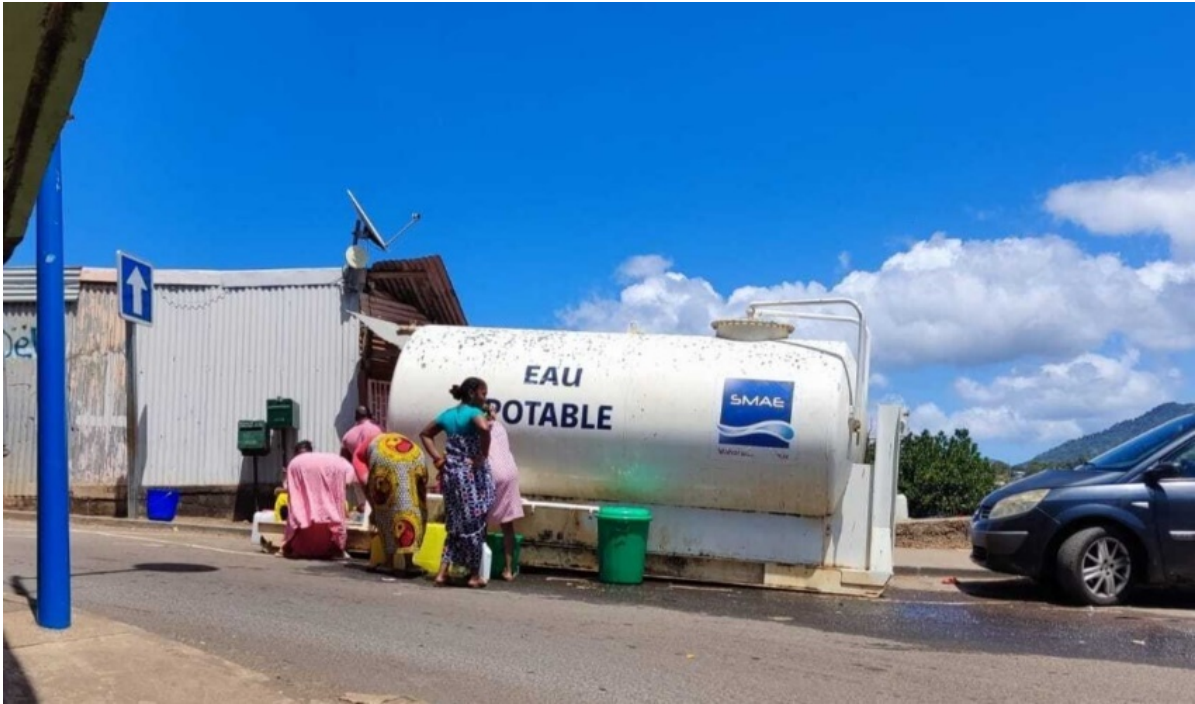
Figure 2. Tank with drinking water - M'tsapere (August 31, 2023)
