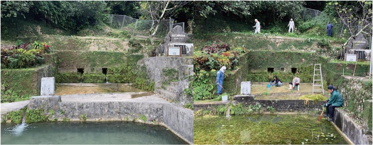
Figure 3. Yan gā on Miyagi Island. Left: an example of a traditional kō where the water basin, stonework, channels, and access space remain visible. Right: community members cleaning and maintaining the site. Location shown in Fig. 2 .
