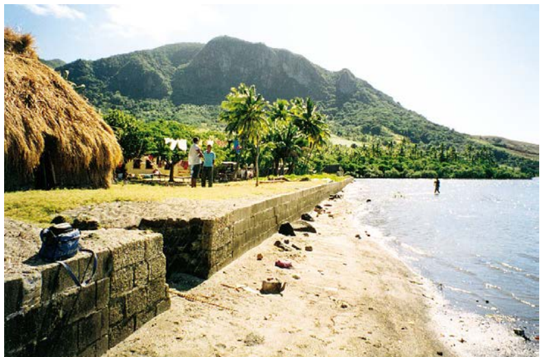
Figure 2: A seawall made out of beach rocks (left) and a seawall made out of concrete (right). From Mimura (1999)
