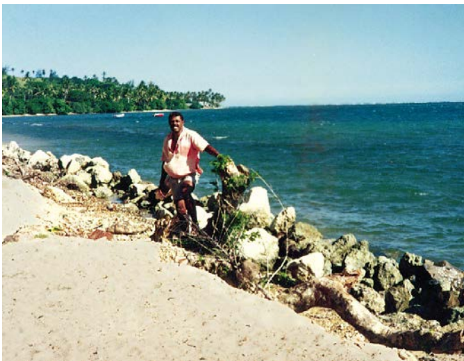
Figure 2: A seawall made out of beach rocks (left) and a seawall made out of concrete (right). From Mimura (1999)
