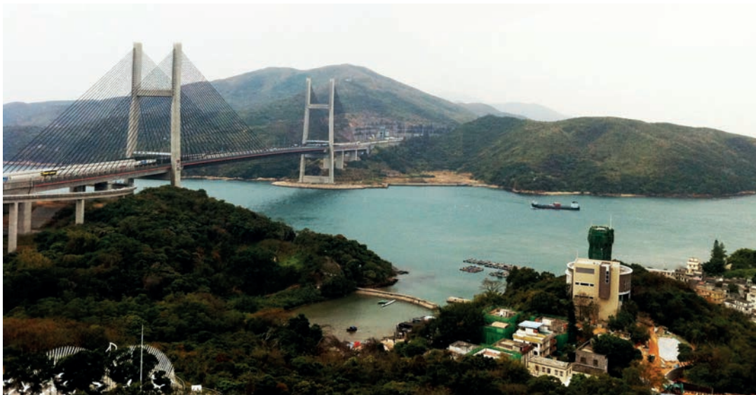
Figure 3: A series of bridges connect the peripheral islands of Lantau Island, Ma Wan, and Tsing Yi to the urban core of Kowloon and Hong Kong (Photo taken at Ma Wan). (Source: © Abraham Leung)
