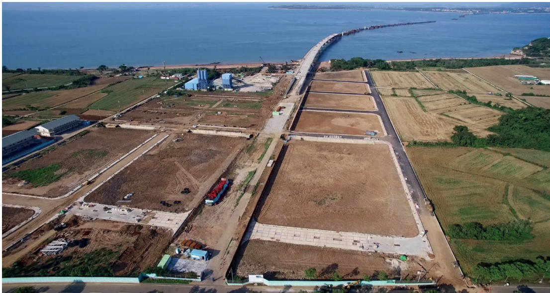
Figure 2: Kinmen Bridge under construction. (© Qing-Zhang Hong, 28 April 2016)
